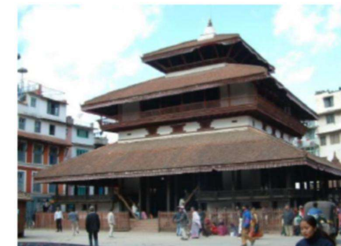
Fig. 1 Kathmandap (pre-2015) before the 2015 earthquake
