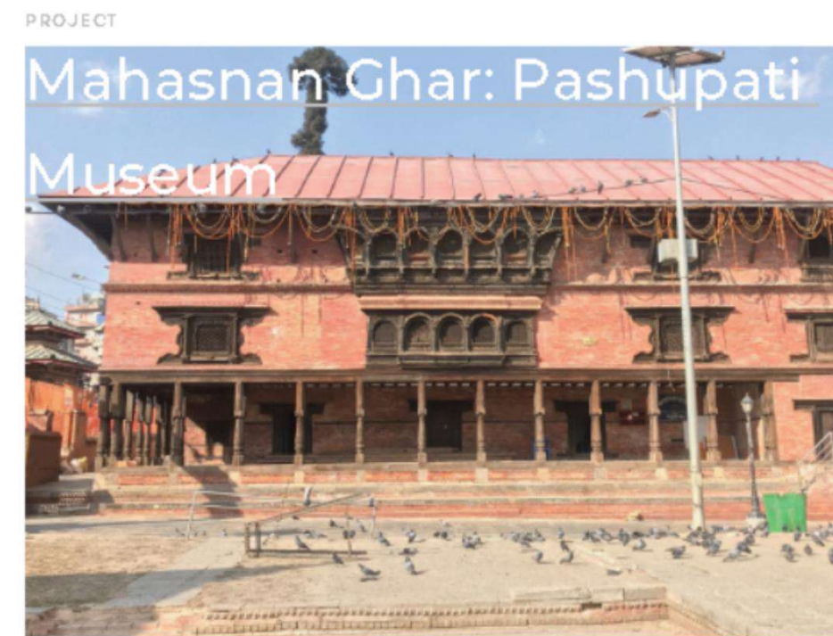
Fig. 1 Southern facade of Mahasana Ghar after the restoration work.
