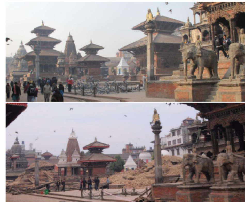
Fig. 1 (A) View of Darbar Square, before and (B) after the earthquake. The two most important temples, Hanuman and Chhatrapati, totally collapsed. Photographs by Rohit Malikar, 2015 and April 26, 2018.
