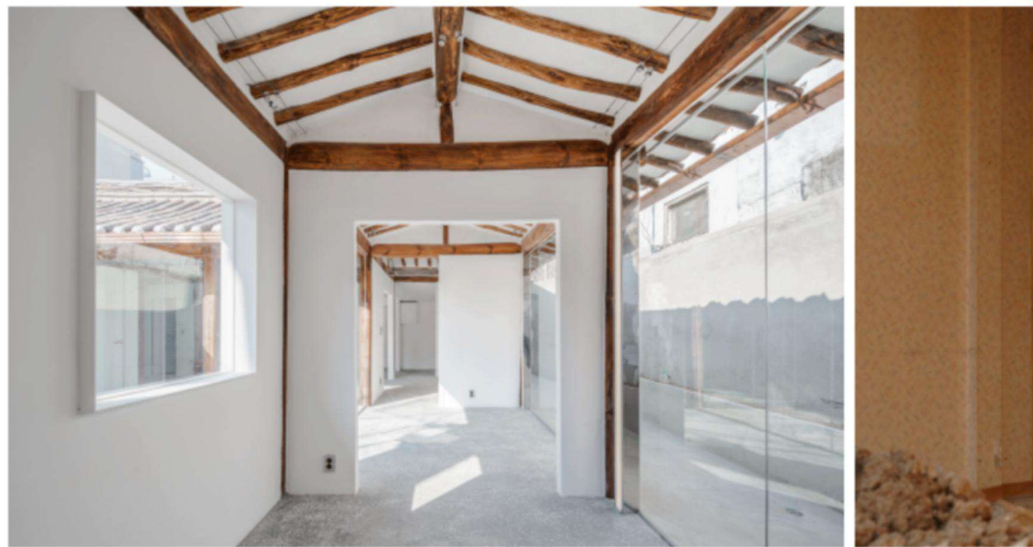
HyeHwa Hanok Renovation 2022
