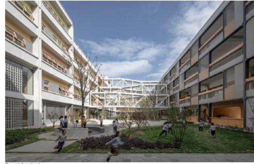
The central courtyard
