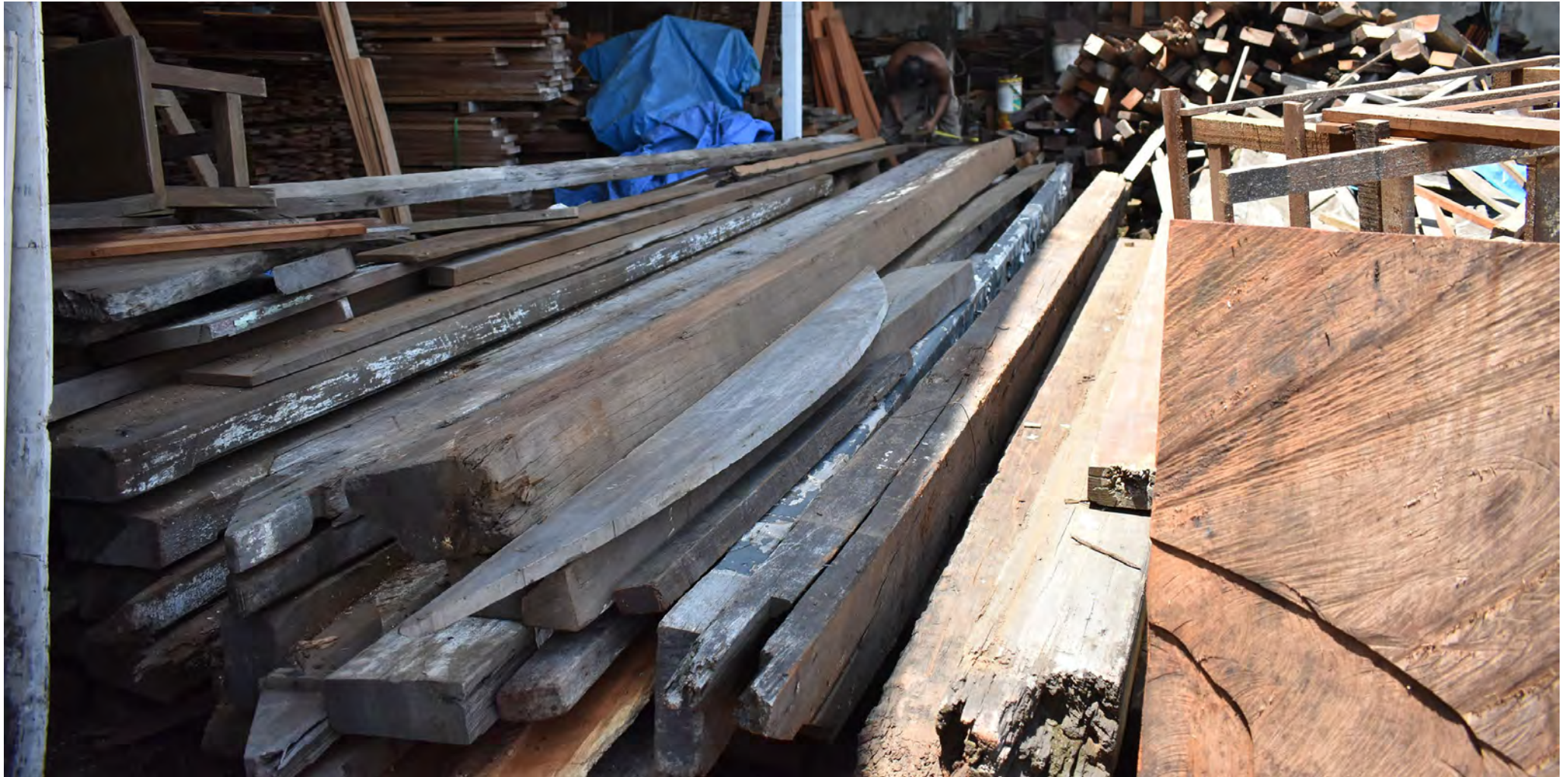
The old wood retrieved from our site were laid in the workshop for measurements and sorting. Timber planks of similar types and tones taken down from other buildings were also being selected to be used for the project since the quantity retrieved from our demolished building was inadequate.
