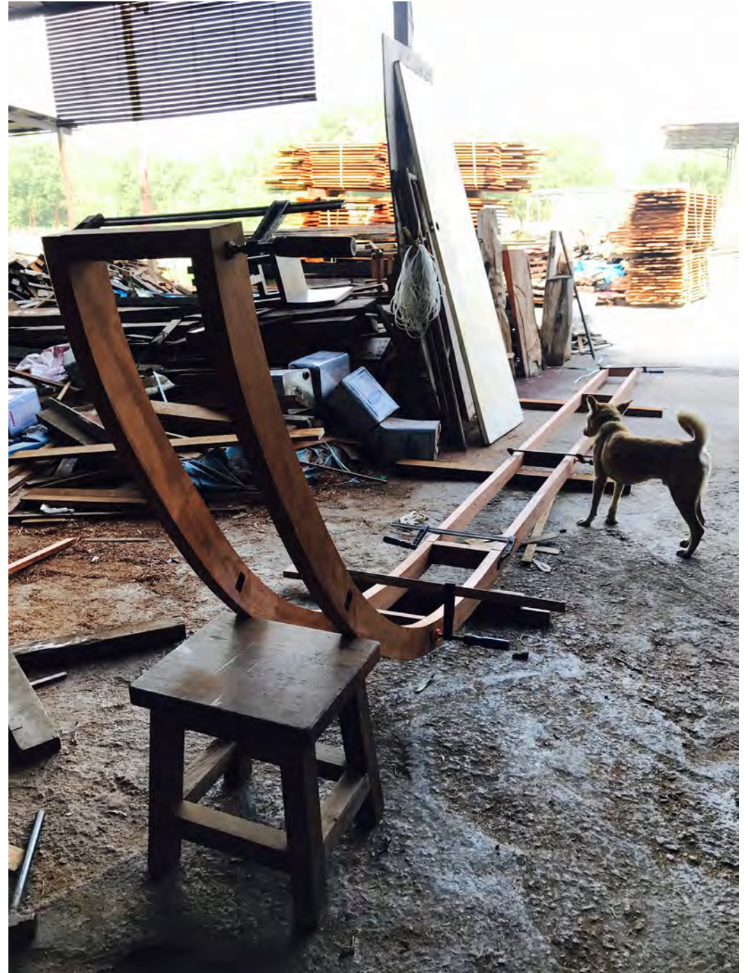
1:1 mock up of the timber facade
