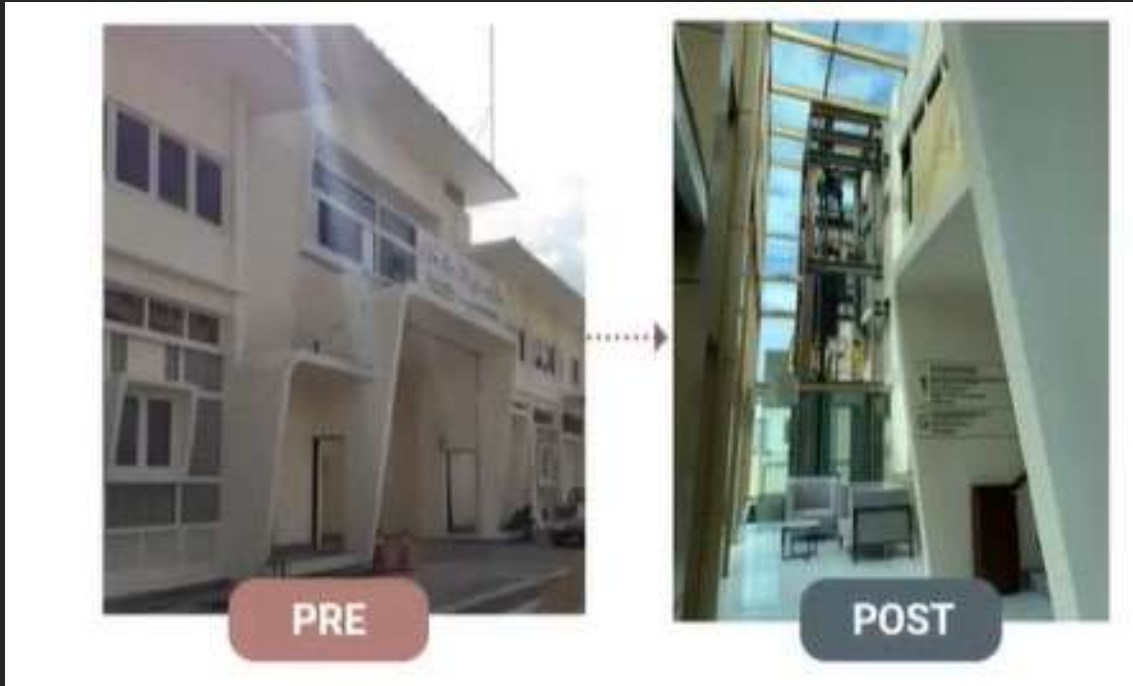
WINDOW BLOCK BEFORE AND AFTER RESTORATION
