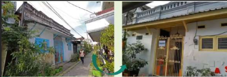
ASRI INN BEFORE AND AFTER RESTORATION
