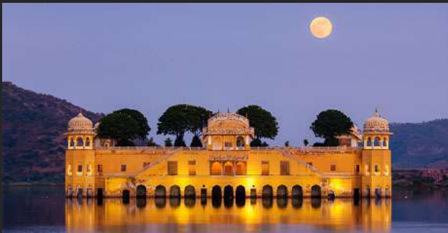
BEFORE-AFTER RESTORATION OF JAL MAHAL
