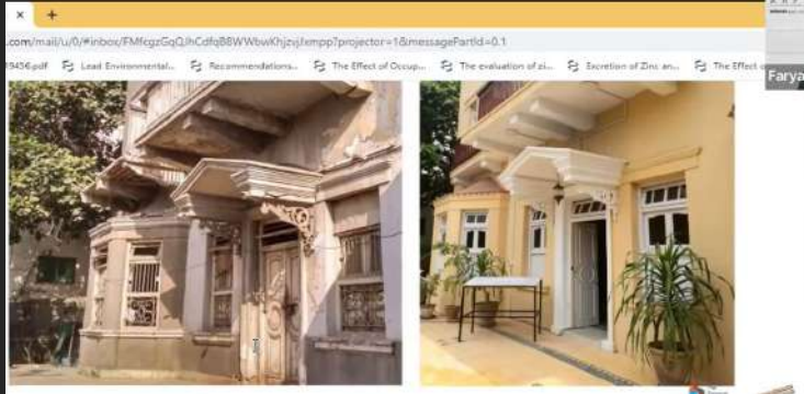
TDF GHAR EXTERIOR BEFORE AND AFTER RESTORATION
