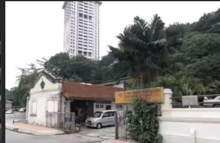
ADJACENT LOT BEFORE RESTORATION
