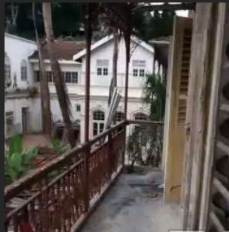
LOKE HOTEL VERANDA BEFORE RESTORATION
