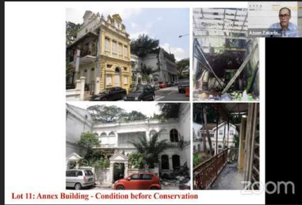
Lot 11: Annex Building - Condition before Conservation
