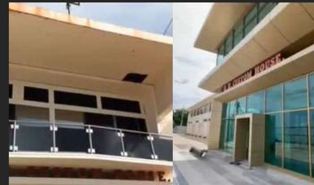
SIGNAGE BEFORE AND AFTER RESTORATION
