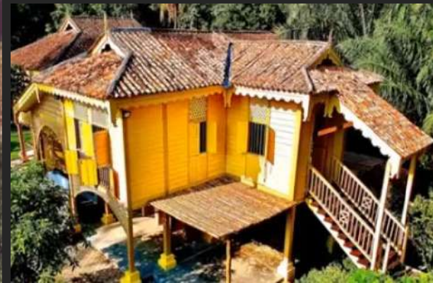
RUMAH KUNING HOUSE BEFORE AND AFTER RESTORATION
