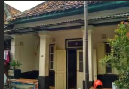
ONGKO LORO HOUSE BEFORE AND AFTER RESTORATION
