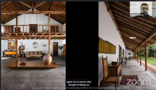
HORAGOLLA HOME AFTER RENOVATION THAT WAS PREVIOUSLY USED AS A STABLE
