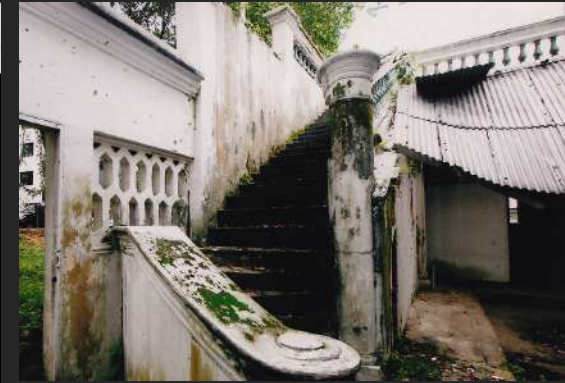
LOKE HOTEL STAIR BEFORE RESTORATION
