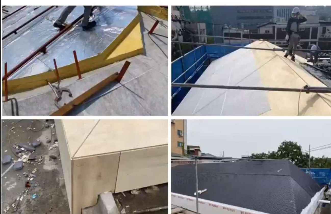
REMOVAL OF THE PREVIOUS ROOF FOR THE NEW INSTALLATION WITH RAINWATER AND DAMPROOFING STRATEGIES
