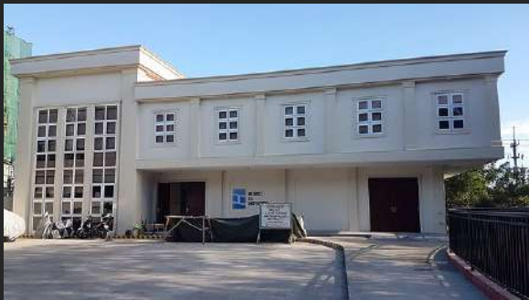
ANCILLARY BUILDING AND INTERIOR AFTER RESTORATION
