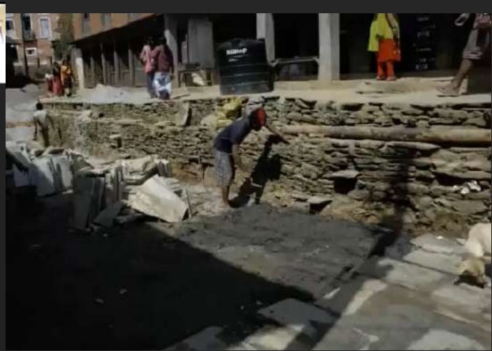
DURING PAVEMENT RESTORATION
