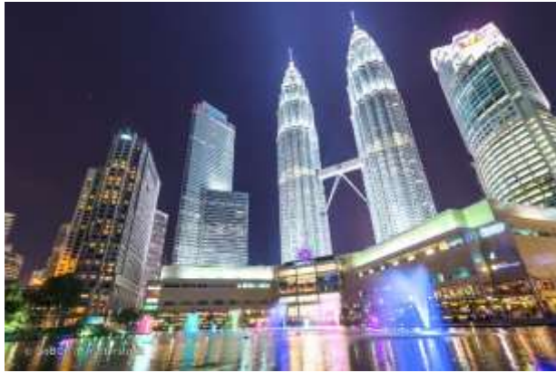
PETRONAS TWIN TOWERS
