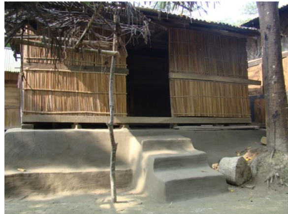
Figure 1 One type of many indigenous houses in Bangladesh: wood frame, mud floor, wall of wood strips, and CI sheet roof at Sutiakati, Swarupkati,
