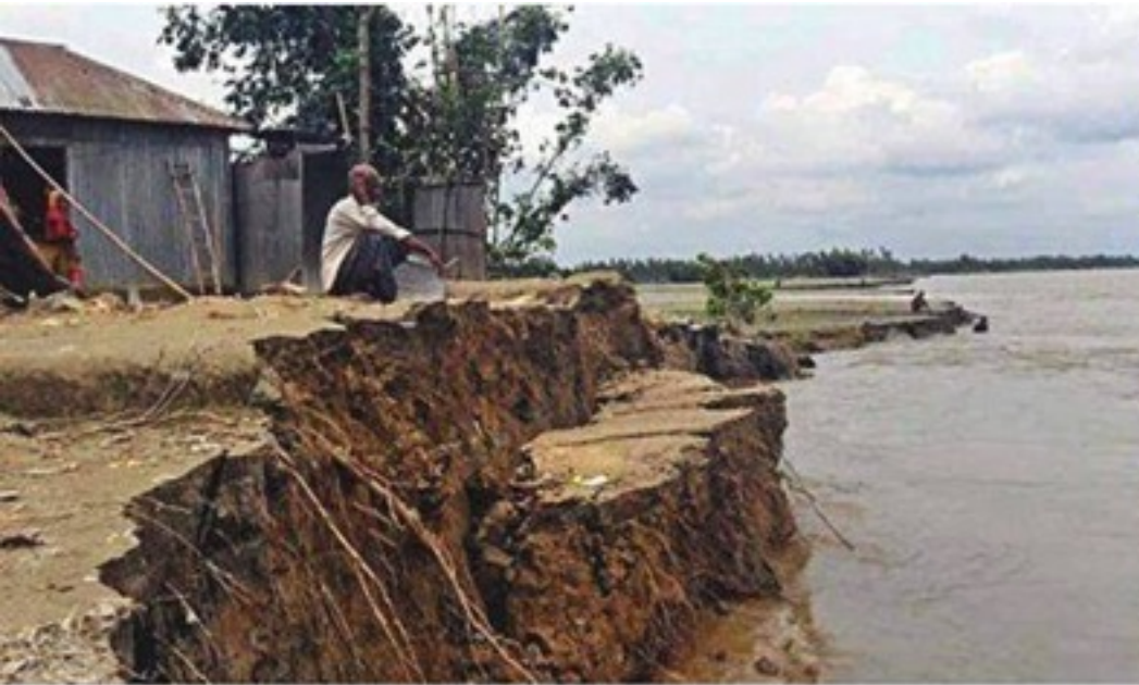
DEVASTATION DUE TO RIVERBANK EROSION
