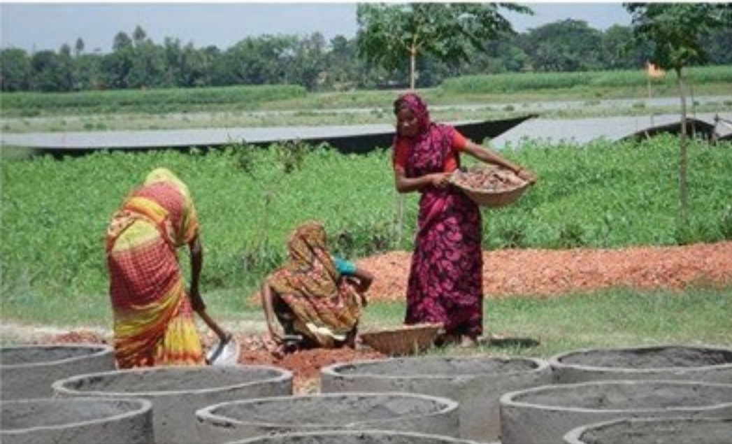
WOMEN IN CONSTRUCTION WORK OF RING PITS
