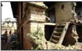
then using traditional heavy materials like brick, cement, wood, steel, etc.
