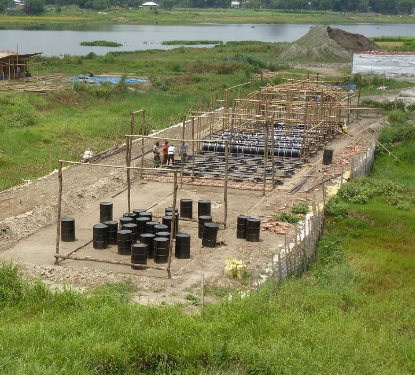
Substructure work in progress.
