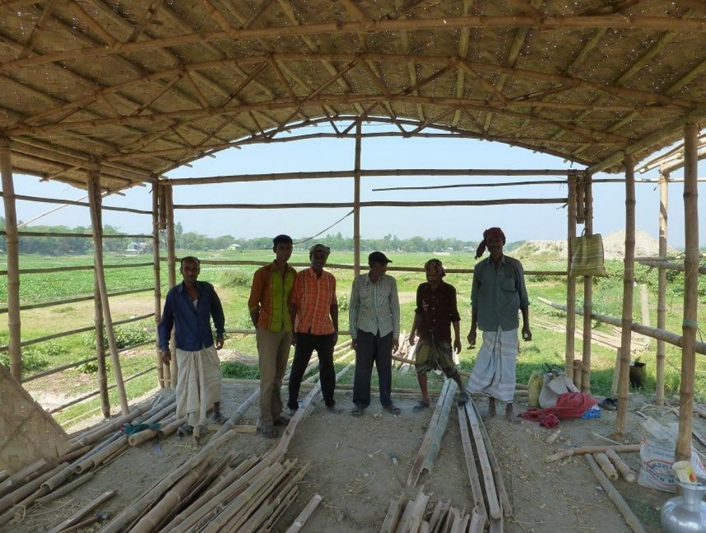
Roof of the mock up installed.
