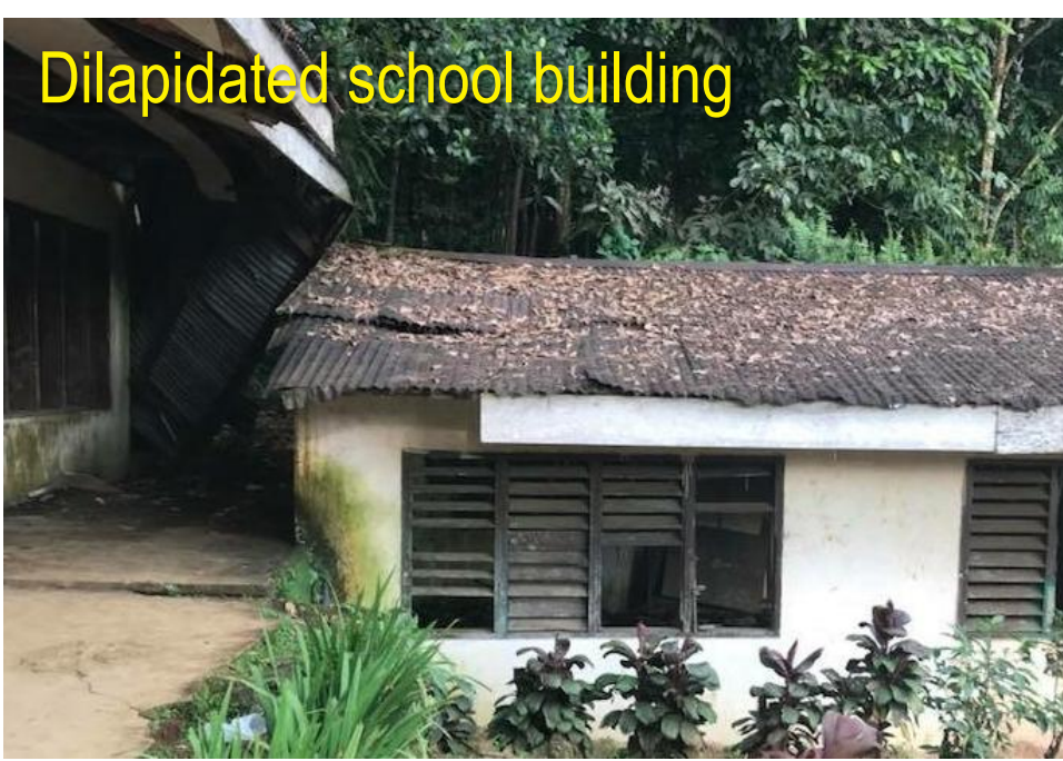
Damaged roofing
