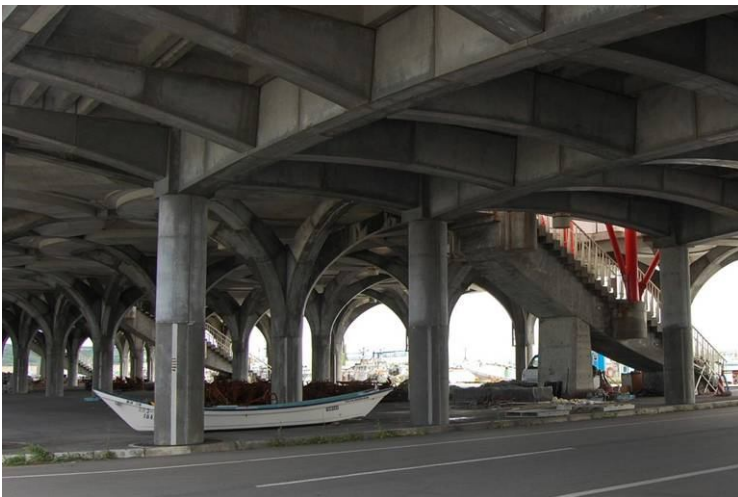
Emergency evacuation facility at sea side
