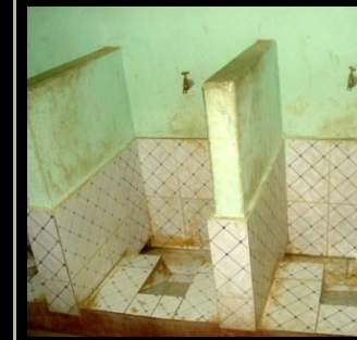
Thick partition wall?
