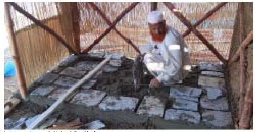
Household members mixing mortar and discussing stone for foundation
