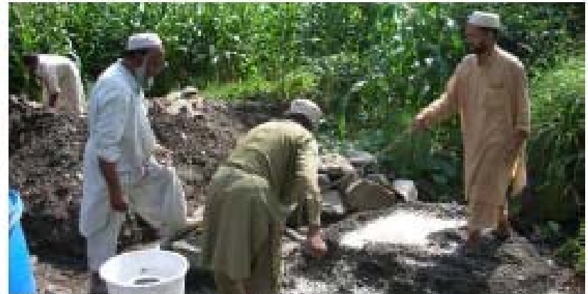
Household members mixing mortar and discussing stone for foundation
