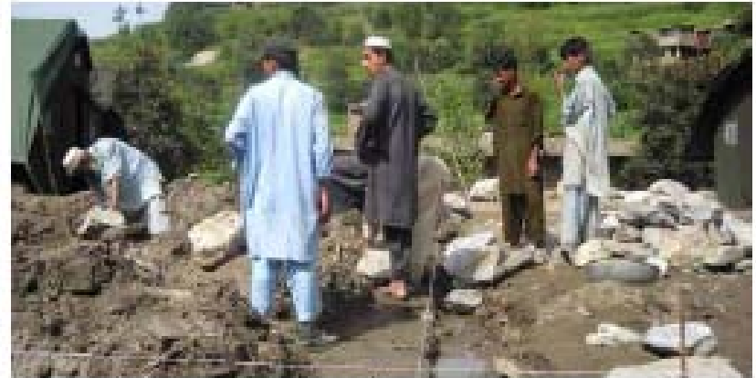
Community members assist in the construction of foundation and laying path
