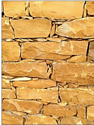
EXPOSED RANDOM RUBBLE MASONRY IN EXTERIOR WALLS
