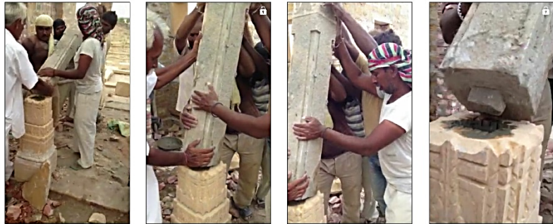
FIXING OF STONE PILLAR
