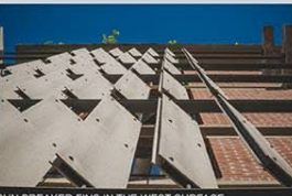
SUN BREAKER FINS IN THE WEST SURFACE
