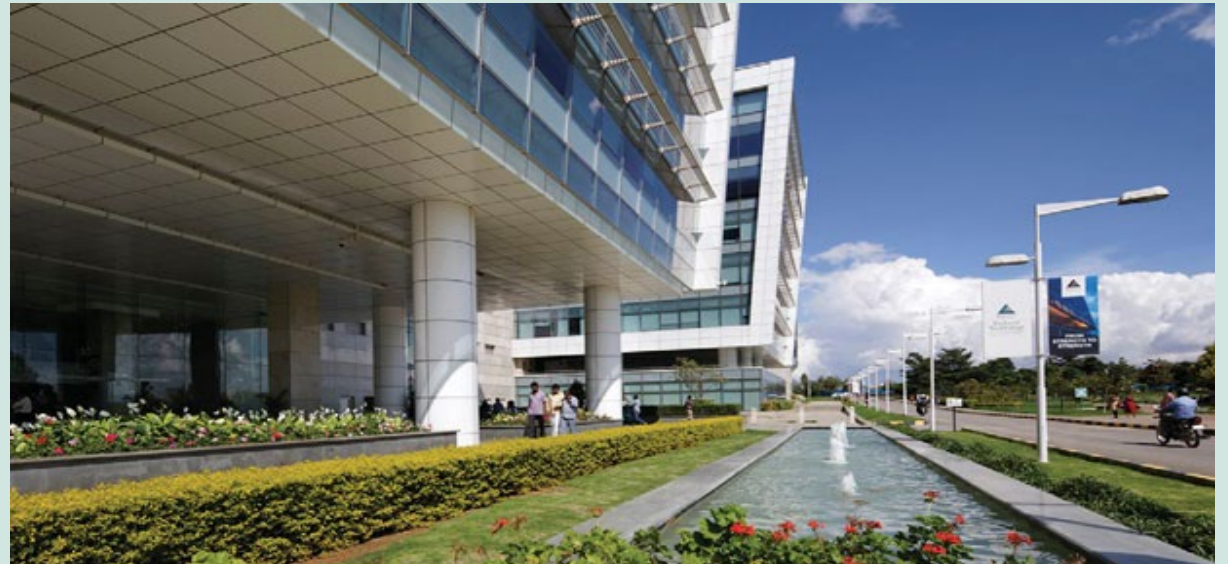
Embassy Tech Village- IGBC Platinum
