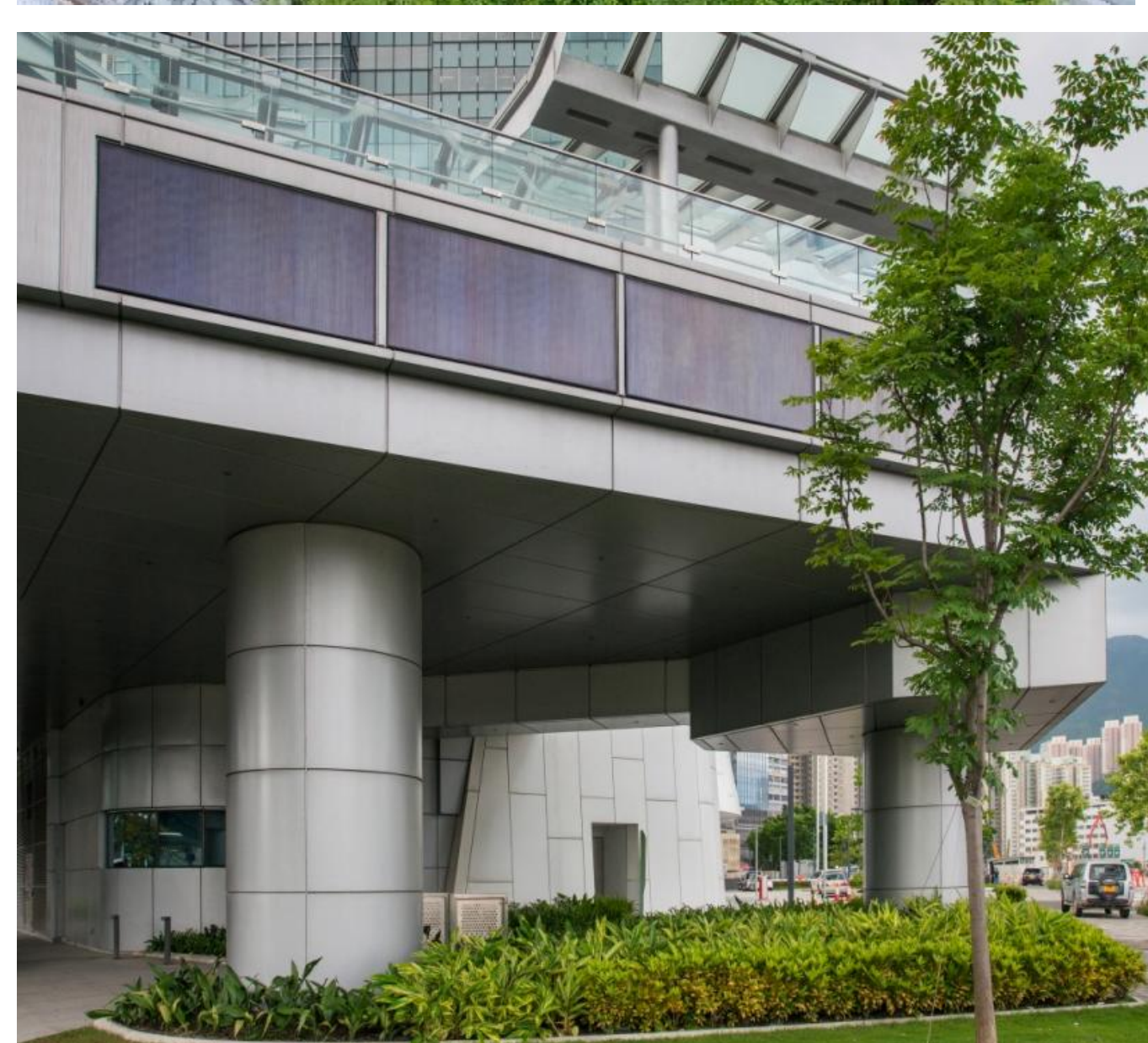
Solar hot water panel in external landscaped area
