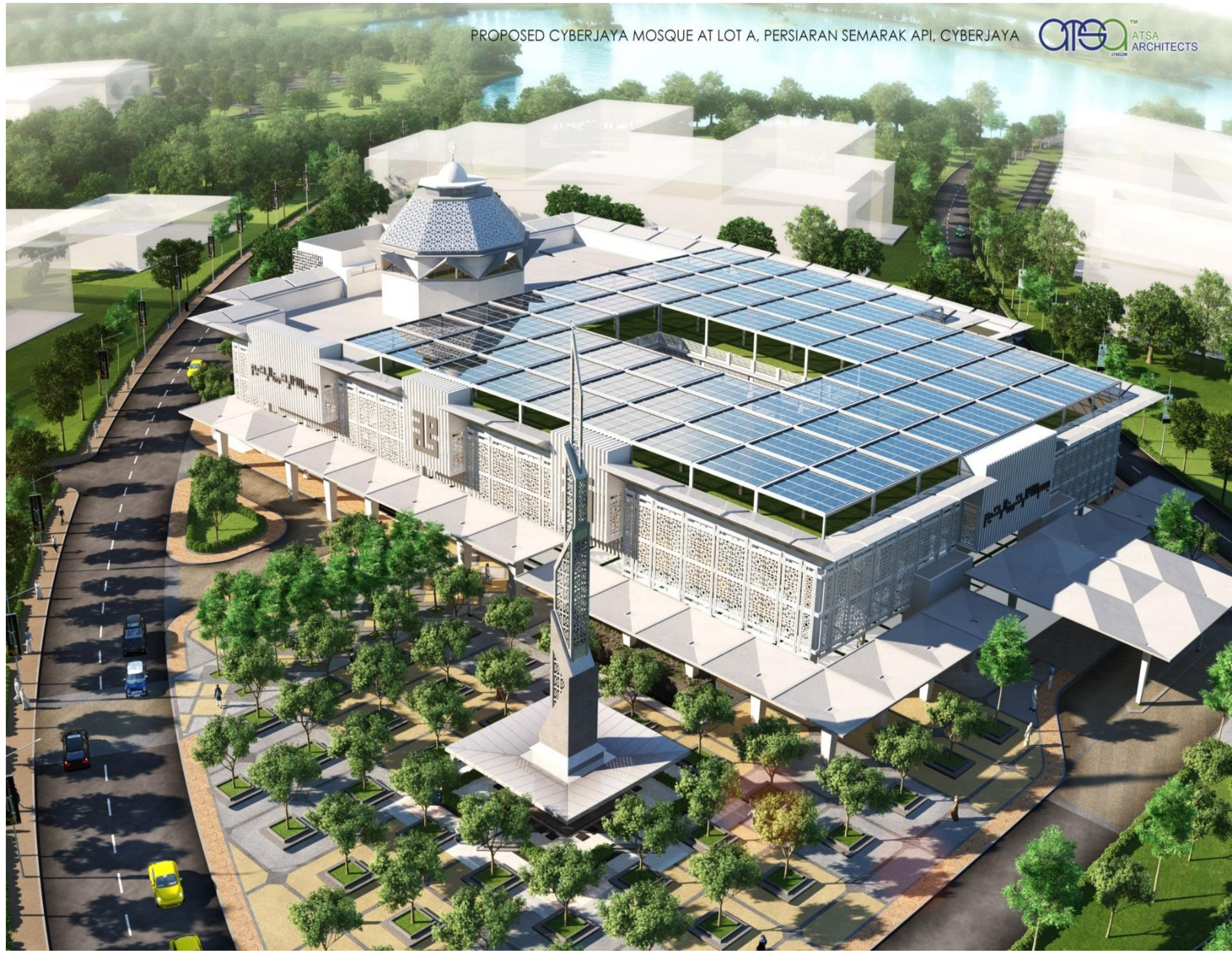
The energy generated from the mosque's solar panels are also supplied to the national grid, contributing to the country's supply of renewable energy. The mosque's main prayer hall has been designed to be air-conditioned for two hours during Friday prayers and during prayers of other special Islamic occasions.
