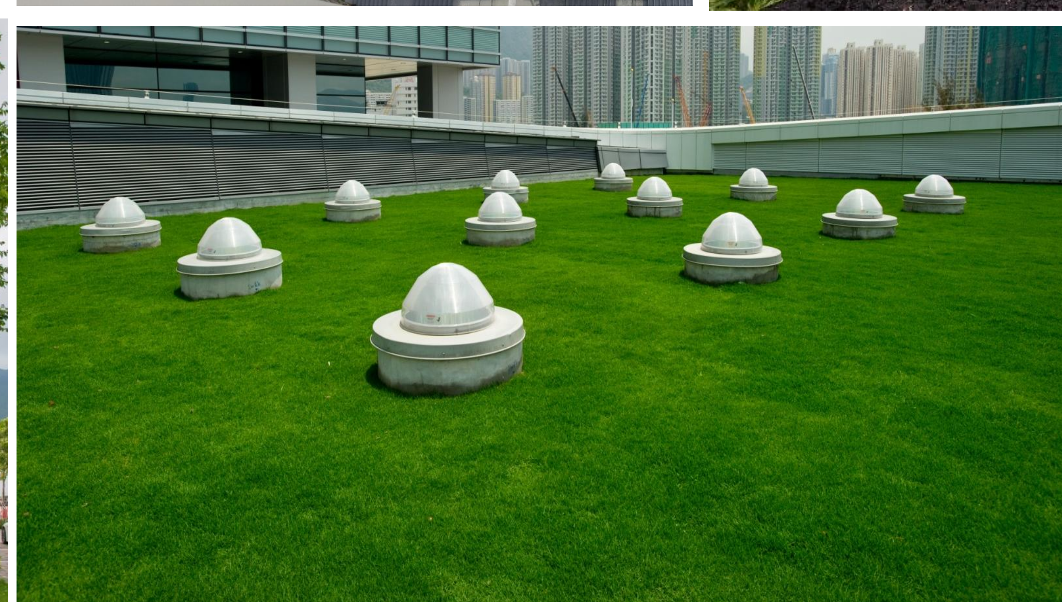
Light pipes in community hall roof for vertical daylight transmission
