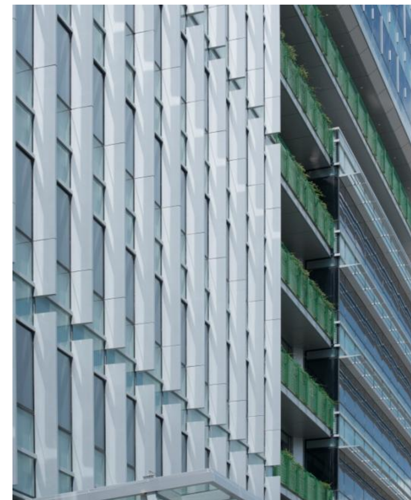
Vertical and horizontal sunshades on facade
