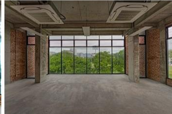
Materials were selected carefully to reflect the client's intention to keep the building as "raw" as possible.
