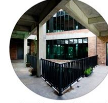
Carved Out Central Courtyard allows daylight to reach most office spaces; Nako Windows made cross and stack ventilation possible
