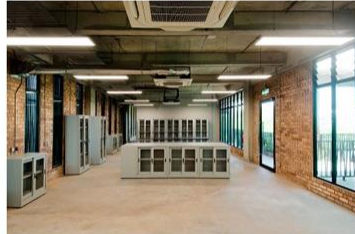
Nako windows were installed at high levels of all office spaces for natural cross & stack ventilation through the central courtyard.
