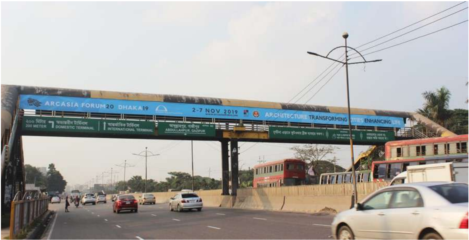
Foot over bridge banners
