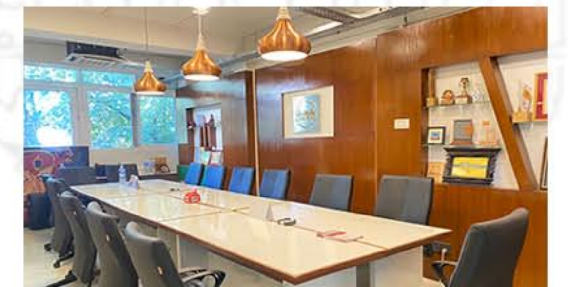
SONA Office renovation
