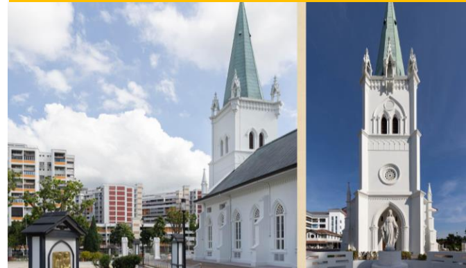
4219 - Restoration and Alteration/Addition Works to existing Church of the Nativity of the Blessed Virgin Mary (Singapore)
